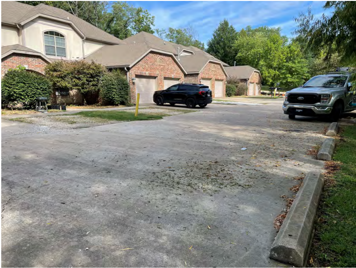
Figure 1: Site photo of existing drive (S Grace Ave).
